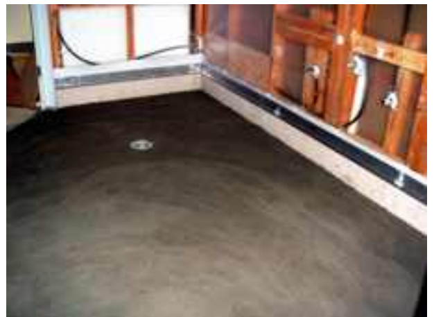
NEW TOPPING WITH 1:60 GRADE TO NEW FLOOR WASTE
