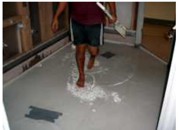
NEW TOPPING WITH 1:60 GRADE TO NEW FLOOR WASTE
