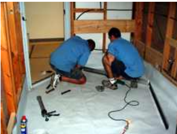
SLIP SHEET & REINFORCING MESH INSTALLED
