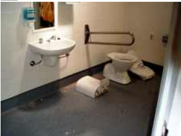
✓ NEW PAN IS INSTALLED
